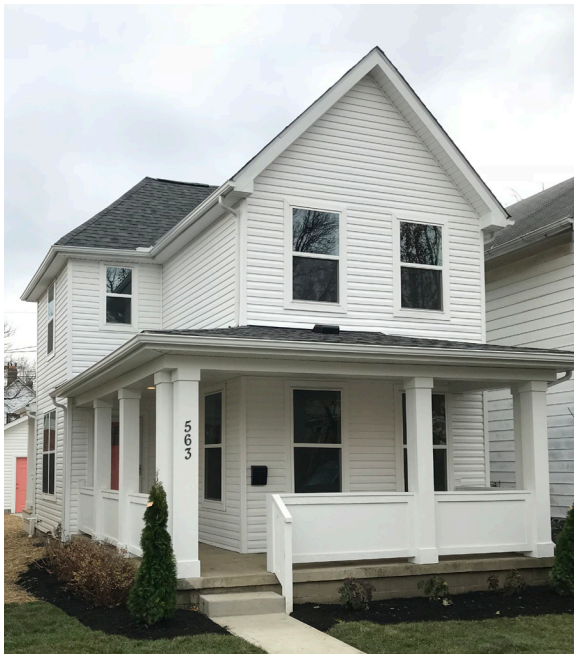
Neighborhood home after rehab of a neglected property.
