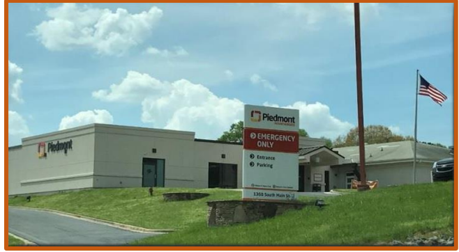
Piedmont Mountainside Hospital Emergency Services
